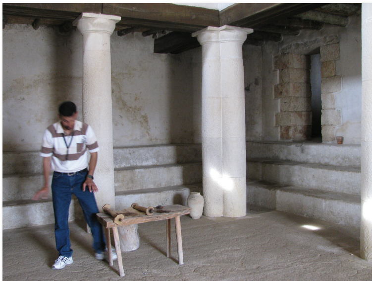
In the synagogue, a building used not only for worship, but as a town hall and courthouse, the Scriptures are read. The Law (Torah), the Prophets, as well as probably legal documents were generally kept in a room off to the side, shown here in the upper right of the photograph.
