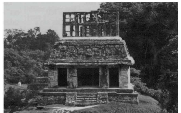
Temple of the Sun. All of the buildings originally had the same floor plan, an outer court and an inner sanctuary. The Temple of the Sun is the best preserved of the three buildings.
